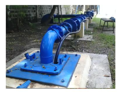
Figure 8 Typical Submersible Pump in PWs
