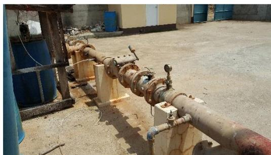
**Photo 17: Production Well #24 Meter Assembly**
