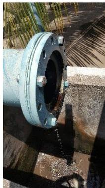
**Photo 34: Water Dripping at Flushing Line**
