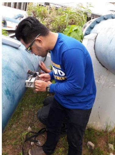
**Photo 44: Actual Installation of Clamp-on Ultrasonic Meter at Macasandig Old Booster Bank #1 Meter**
