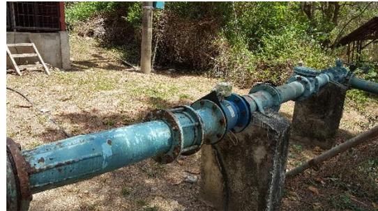
Photo 10: Production Well #18 Meter Assembly
