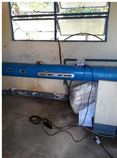
**Photo 46: Actual Installation of Clamp-on Ultrasonic Meter at Production Well #5 Meter**
