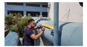
Photo 35: Actual Installation of Clamp-on Ultrasonic Meter at Macasandig Old Booster Bank #1
