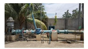
Photo 32: Production Well #29 Supply Meter Assembly
