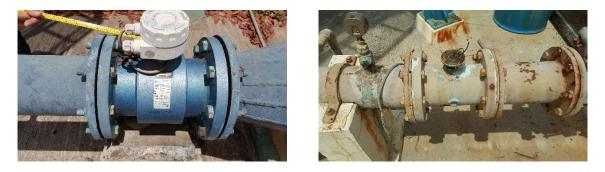
Photo 4: No Converters/Displays (PW #15 and #24)
