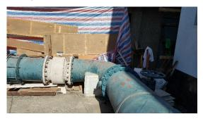
Photo 39: Macasandig New Booster Supply Meter Assembly
