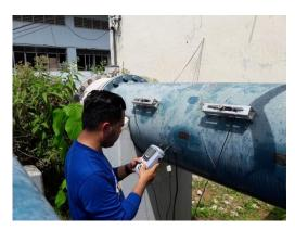
Photo 45: Actual Installation of Clamp-on Ultrasonic Meter at Macasandig Old Booster Bank #2 Meter
