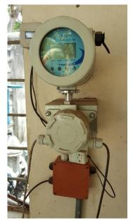
Photo 15: Production Well #10A Converter (Blackout Display)
