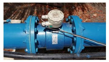
Photo 2: No Conduit and Grounding System (PW #10A)
