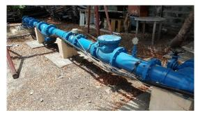
Photo 14: Production Well #10A Meter Assembly
