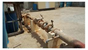
Photo 17: Production Well #24 Meter Assembly
