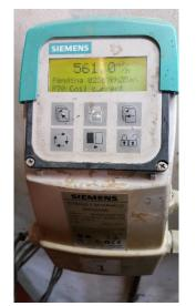
Photo 6: F70 Coil Current Fault Alarm at Macasandig Old Booster Bank #1
