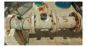
Photo 16: Production Well #24 Supply Meter (Detached Converter)
