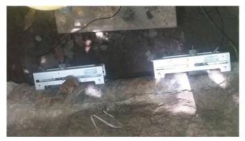
Photo 41: Actual Installation of Clamp-on Ultrasonic Meter at Carmen Line
