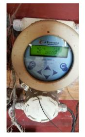
Photo 3: Fading Digital Segments (PW #18)
