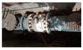
Photo 20: Balulang Booster (Bulua Line) Supply Meter
