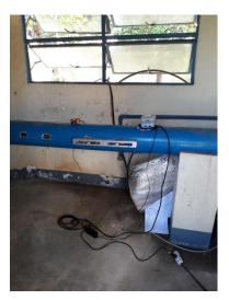
Photo 46: Actual Installation of Clamp-on Ultrasonic Meter at Production Well #5 Meter
