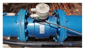
Photo 13: Production Well #10A Supply Meter
