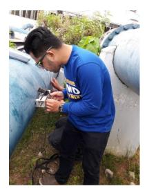
Photo 44: Actual Installation of Clamp-on Ultrasonic Meter at Macasandig Old Booster Bank #1 Meter
