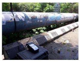
Photo 43: Actual Installation of Clamp-on Ultrasonic Meter at Bugo Booster Line Meter
