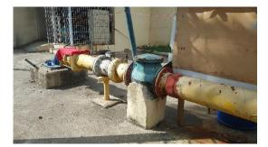
Photo 28: Production Well #23 Supply Meter Assembly
